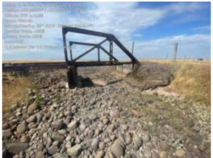
TH002756.JPG 32: 16 ft between pier and abutment on right
