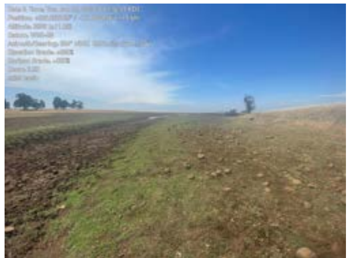
TH002826.JPG 102: exist basin
