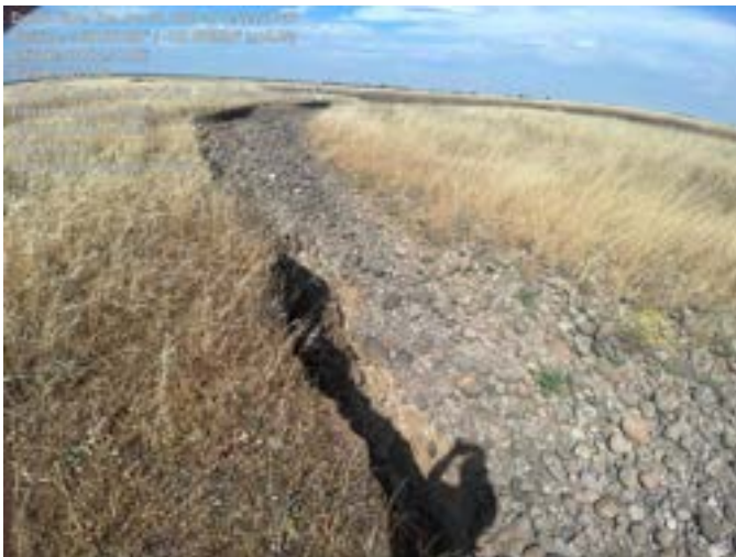
TH002813.JPG 89: bank erosion channel 10 wide
