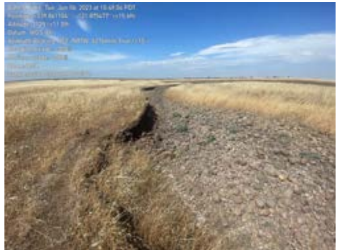
TH002812.JPG 88: bank erosion channel 10 wide
